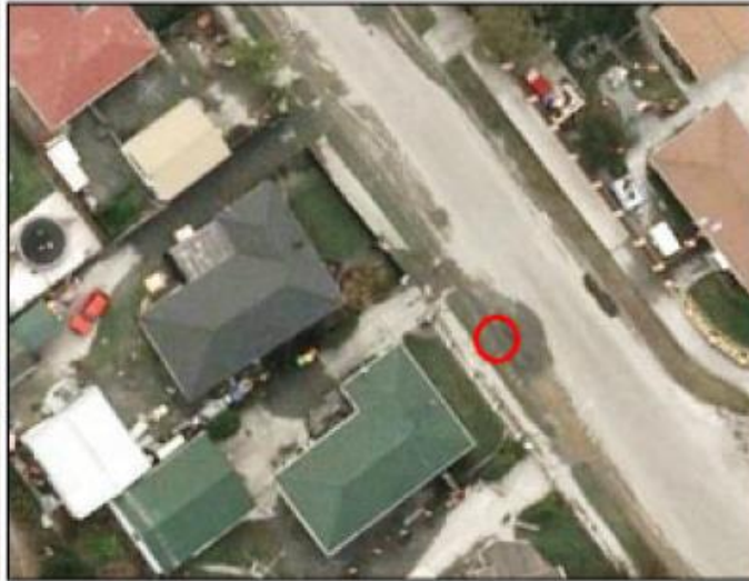
(b) Moderate Liquefaction
